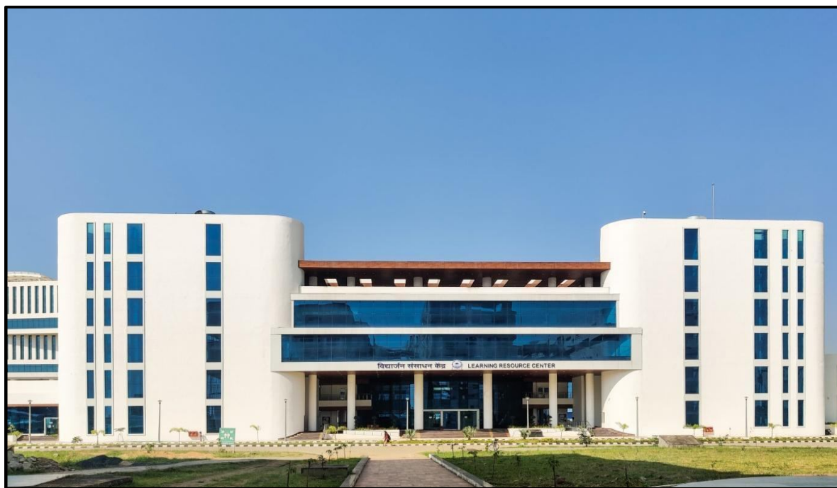
Figure 1. The Learning Resource Center (LRC) Building
